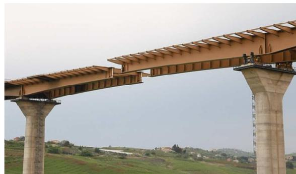
**Fig. 9:** Varo carpenteria metallica
