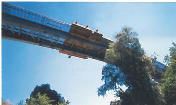
Photo 11 : Outil mobile coffrant / Mobile formwork for the deck slab
